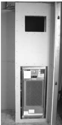
Figure 11: Install chassis centered
